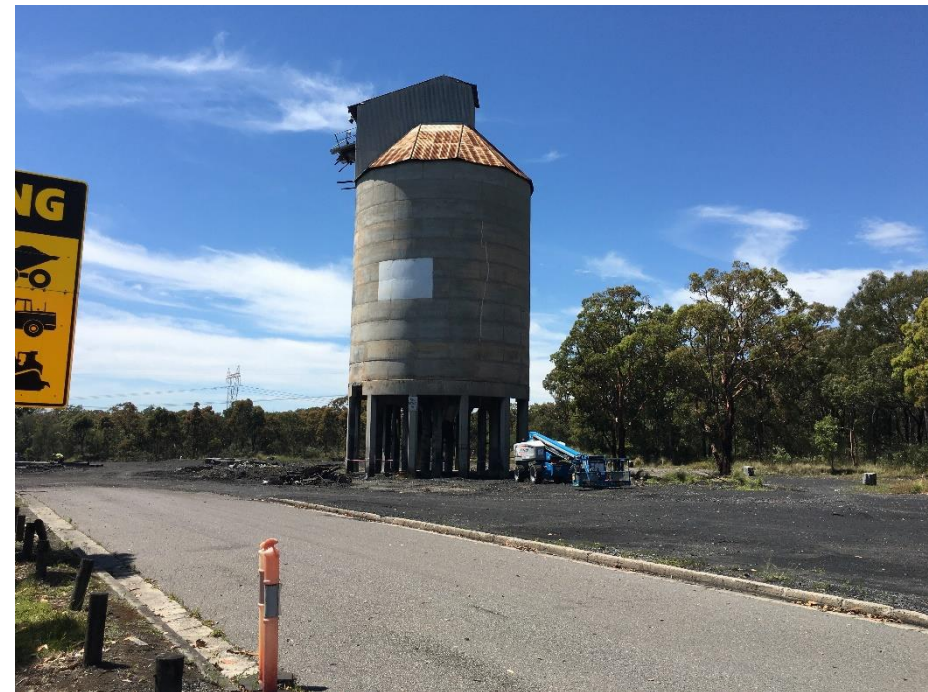
CVC Coal Storage Bin to be demolished
