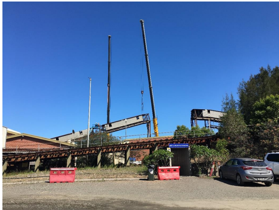
Removal of Back-Drift Gantry
