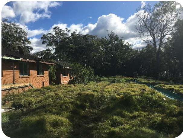
Mine Cottages Demolition July 2020
